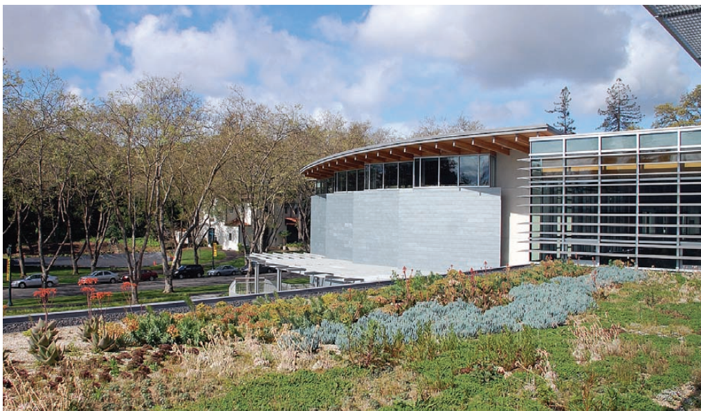
Figure 40 Mills College: Living Roof on the Lorry I. Lokey Graduate School of Business
